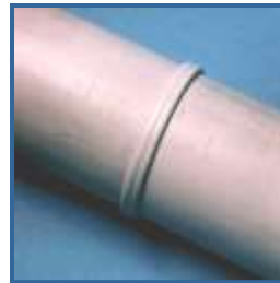
Fig 1- Butt weld
